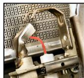
*For the sake of this technical bulletin, the ignitor rod has been painted an orange color. This will allow you to see the exact positioning in accordance with the instructions.*
