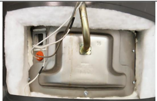
7. Initiate unit operation with the gas turned OFF and verify that igniter is sparking to the pilot hood. Turn gas back ON.
