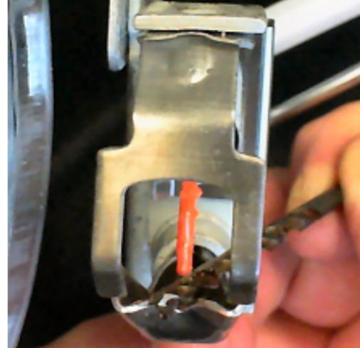
5. The igniter rod should be positioned in the bottom and middle of the saddle of the pilot hood as shown here.
